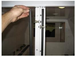
Cut door gasket with utility knife. Cut gasket to the length of door acceptor frame. Attach as shown above.
